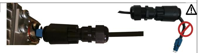
Remove the fiber dust caps from fiber end face and seat into the RRH SPF card slot until you hear a click. Do not twist fiber end face or kink the fiber during installation.
